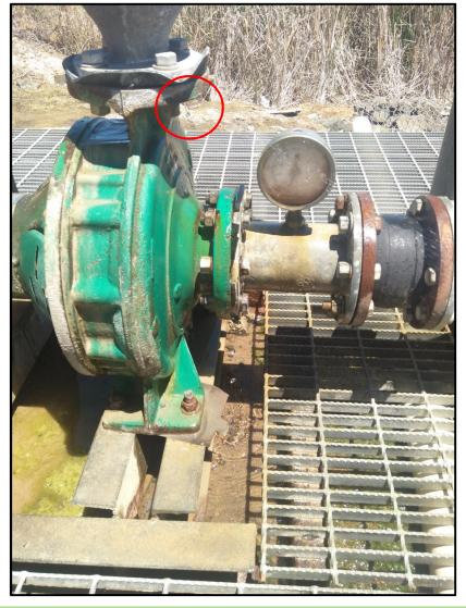
On 4 November 2016 a pump flange adjacent to the Parnells Dam discharge point was observed to have a small pinhole leak. The water accumulated in the discharge point dissipater dam then overtopped the discharge point weir into Parnells Creek.
